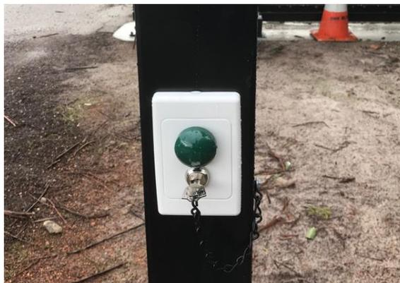
8. If the gate has closed before you operate the key, press the green button above the key switch to re-open the gate.
